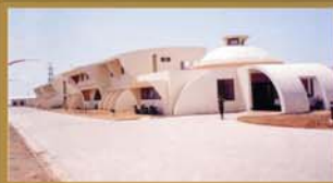
Centre for Wind Energy Technology, Chennai
